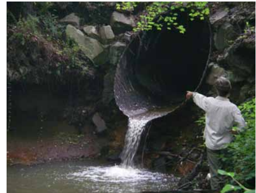
Traditionally engineers managed runoff by channeling it away from homes through large stormwater pipes, sending polluted water flooding into the nearest river.
