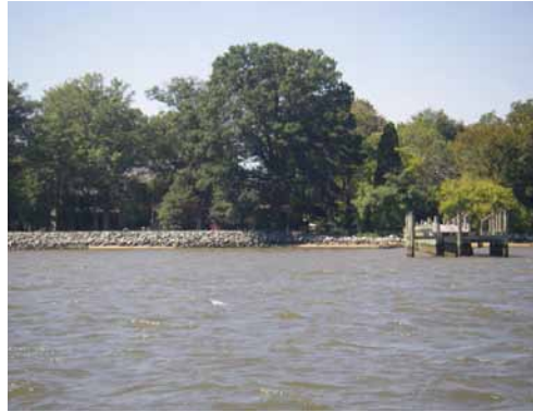
Riprap and other shore-hardening practices increase the force of tides downriver and exaggerate the impacts of storms
