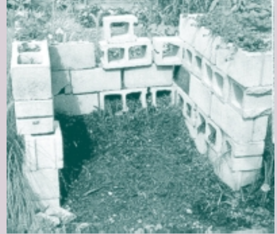
A simple compost bin made of cement blocks.
