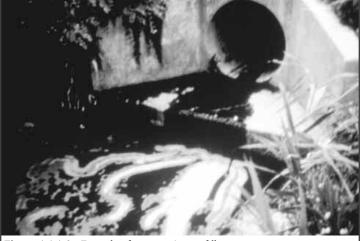
Figure 4.6.4-2. Example of a severe pipe outfall.
