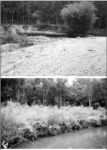
Figure 4.6.3-3. Exposed pipe before and after stream restoration project.
