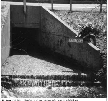
Figure 4.6.5-1. Perched culvert causing fish migration blockage
