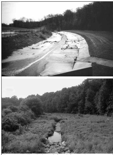
Figure 4.6.1-4. Channelized stream before and after restoration
