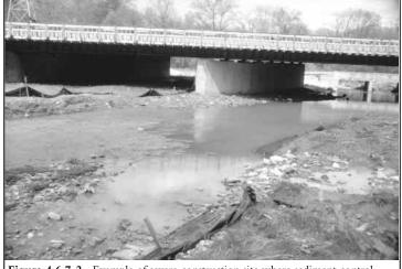
Figure 4.6.7-2. Example of severe construction site where sediment control fencing has failed
