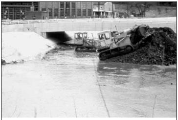
Figure 4.6.7-1. An instream construction site.
