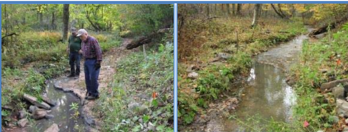
Photos During and Shortly After 2007 CCB-Grout Injection at Hoyes Run. Stream flow was restored within hours of grout injection.
