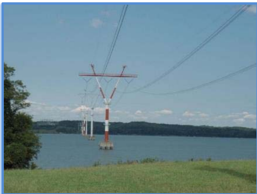
Figure 5-32 Existing 500-kV Transmission Line Crossing of the Potomac River
