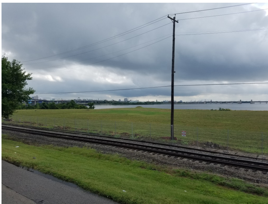
Photo 1: View of site looking northeast. Note small mound of material in center of image.
