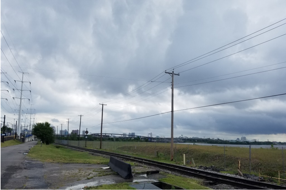
Photo 4: View of mounded material looking northeast.
