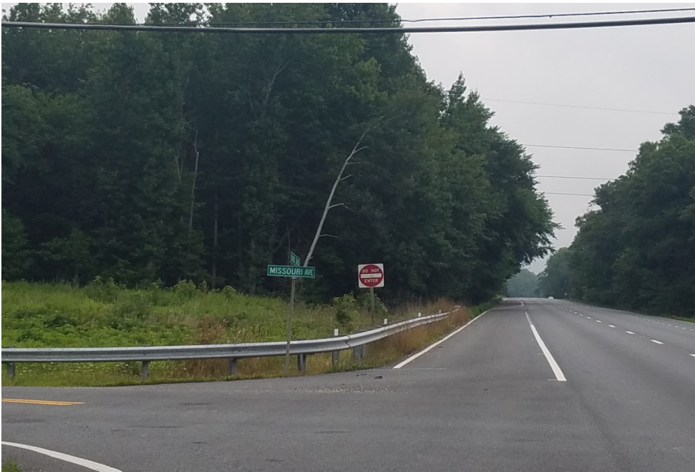
Photo 3: View of Rt. 301 looking northeast from Missouri Ave.
