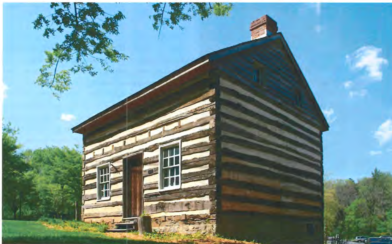
Figure 4.4 The Thomas Isaac Log Cabin is an example of a site that is listed as a Howard County Historic Site and is cared for by the Department of Recreation and Parks.
