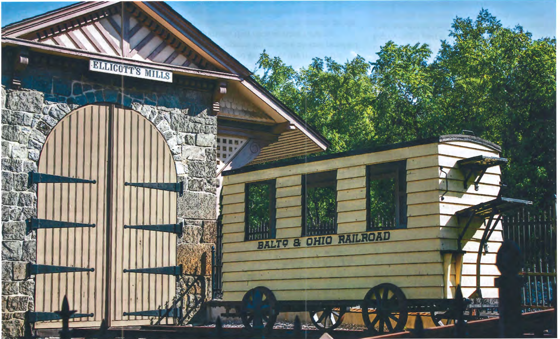
Figure 4.11 Fully acquiring the B & O Ellicott City Station Museum allowed the Living History and Heritage team to increase the number of full time programming and administration positions.
