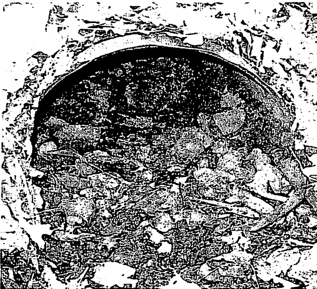
Rusted out culvert.
