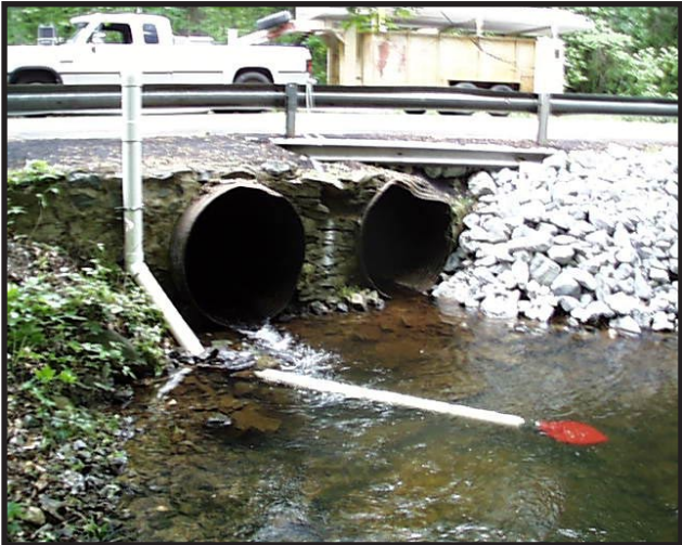
Low Level Strainer Installation
