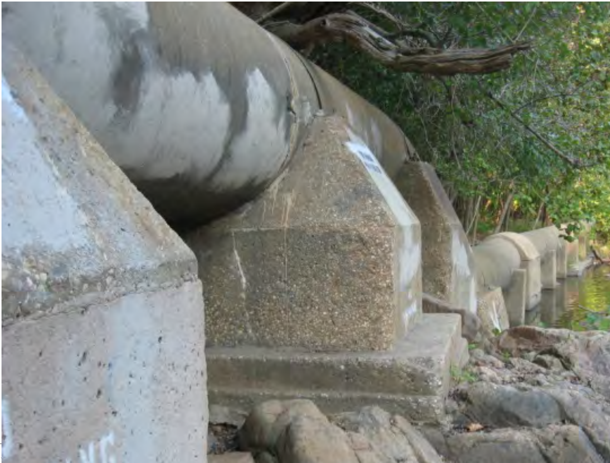
Figure 10- Existing 42-Inch Diameter Sewer.
