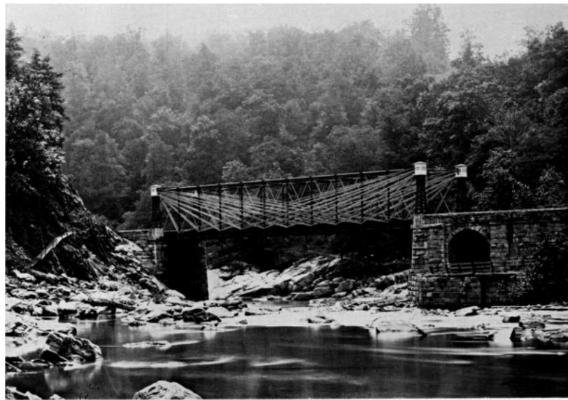
Figure 8 - Pre-dam photo of Railroad Bridge that has been converted to the Grist Mill Trail Cable Stay pedestrian bridge.
