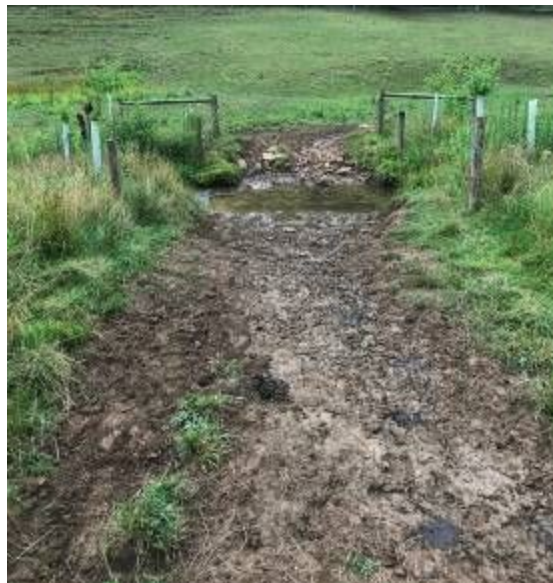
A hardened livestock crossing will be constructed at this site on Little Laurel Run.
