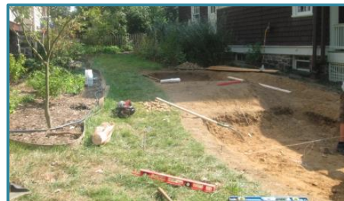
During installation phase
