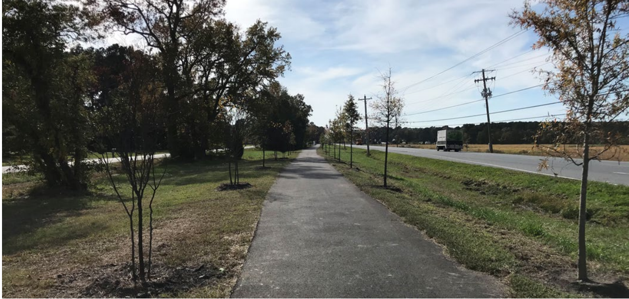
MD-413 Multiuse pathway which provides walking and biking access from Crisfield to Westover in Somerset County.
