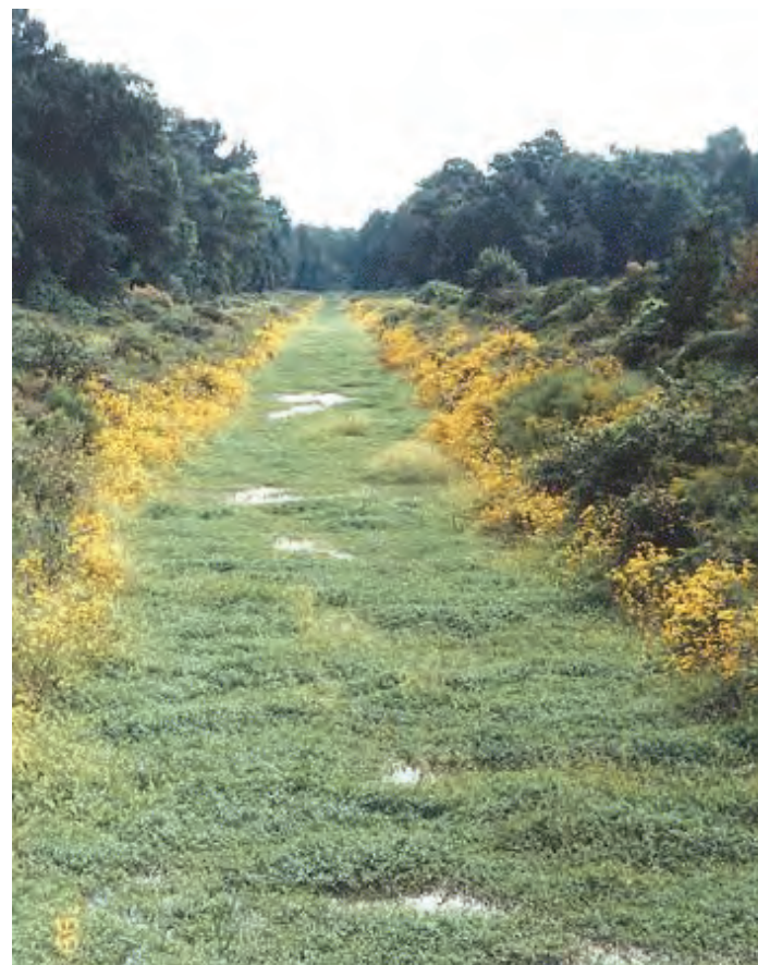
A well-managed drainage system with vegetated channel banks protects soil moisture and water quality.
