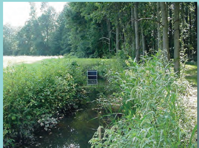
A water control structure built across a drainage ditch prevents gully erosion, reduces nutrient loadings, and controls water levels.
