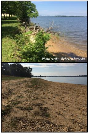
Above: The Conquest Beach Park shoreline is severely eroded and undercut by wind driven waves and boat wakes. Below: Restored shoreline using shingle beach living shoreline design, which mimics natural shorelines and improves resiliency.
