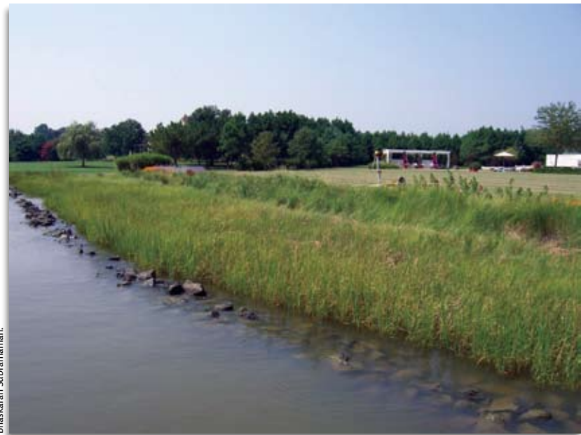
‘Living shorelines’ involve using non-structural shoreline stabilization measures. Living shorelines provide erosion control benefits while also enhancing the natural shoreline habitat. They often allow for natural coastal processes to remain through the strategic placement of plants, stone, sand fill, and other structural and organic materials.
