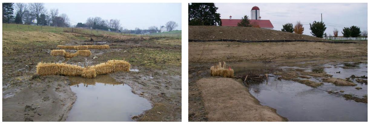
Straw bales to create backwater and increase deposition and reduce further erosion
