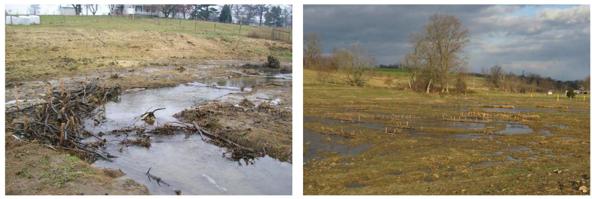
Small woody debris was used to help reduce erosion, collect sediment and more debri
