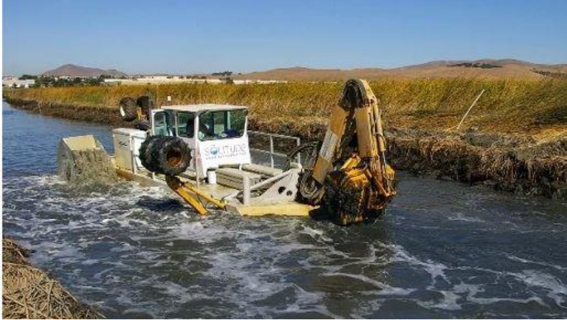
Dredging to increase water depth
