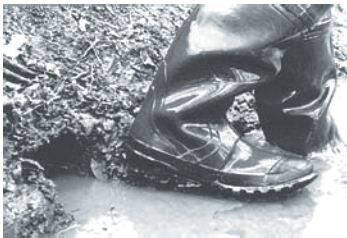
Drive stake in all the way
