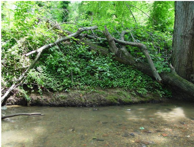
*Figure 10. Suspended log bank protection.*
