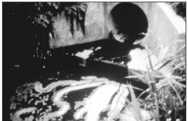
Figure 4.6.4-2. Example of a severe pipe outfall.
