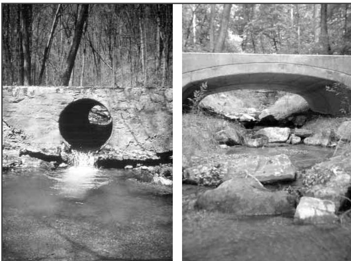
**Figure 4.6.5-4.** Perched culvert before and after restoration project.
