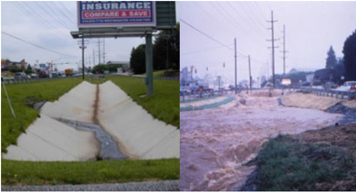
The same drainage before and during a rain event. Large amounts of impervious surface can lead to high flows during even moderate intensity storm events, with several detrimental effects.
