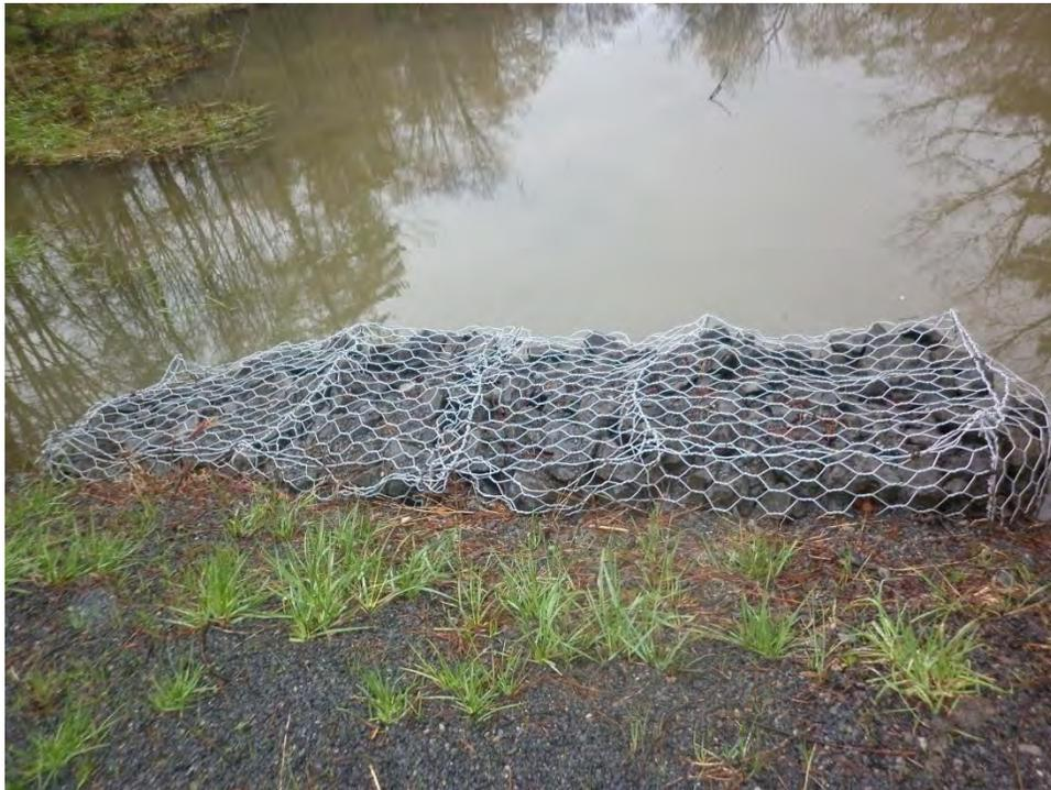
Photo #411 Gabion outlet protection
