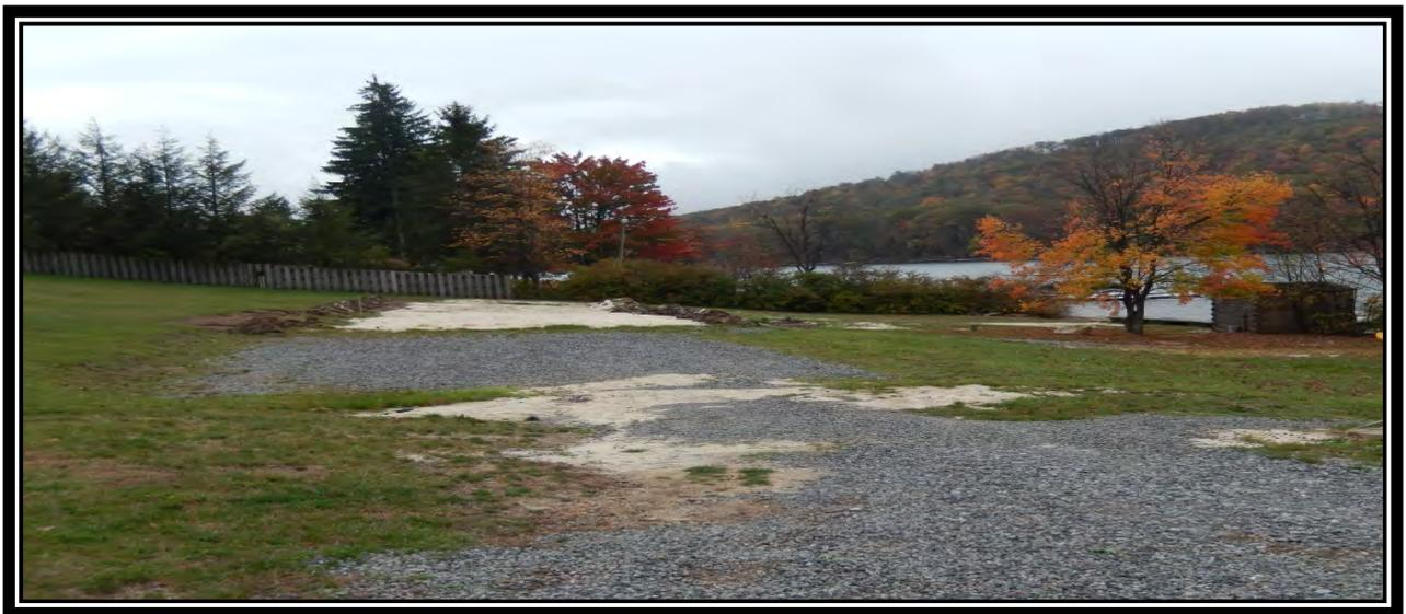
Installation of sand volleyball court, no containment of disturbed soils, directly adjacent to lake
