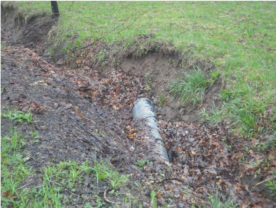
Photo #421 Eroded outfall
