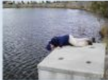
Stormwater BMP Inspections and Repair
