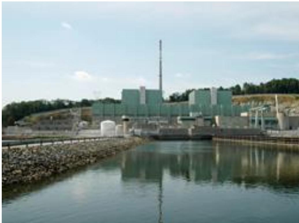
Unit 1 was a 200 MWt, high temperature, gas-cooled reactor that operated from June 1967 to October 1974, when it was permanently shut down. All spent nuclear fuel from Unit 1 was removed from the site, and the Unit 1 spent fuel pool was drained and decontaminated. The Unit 1 reactor vessel, primary system piping, and steam generators remain in place.
