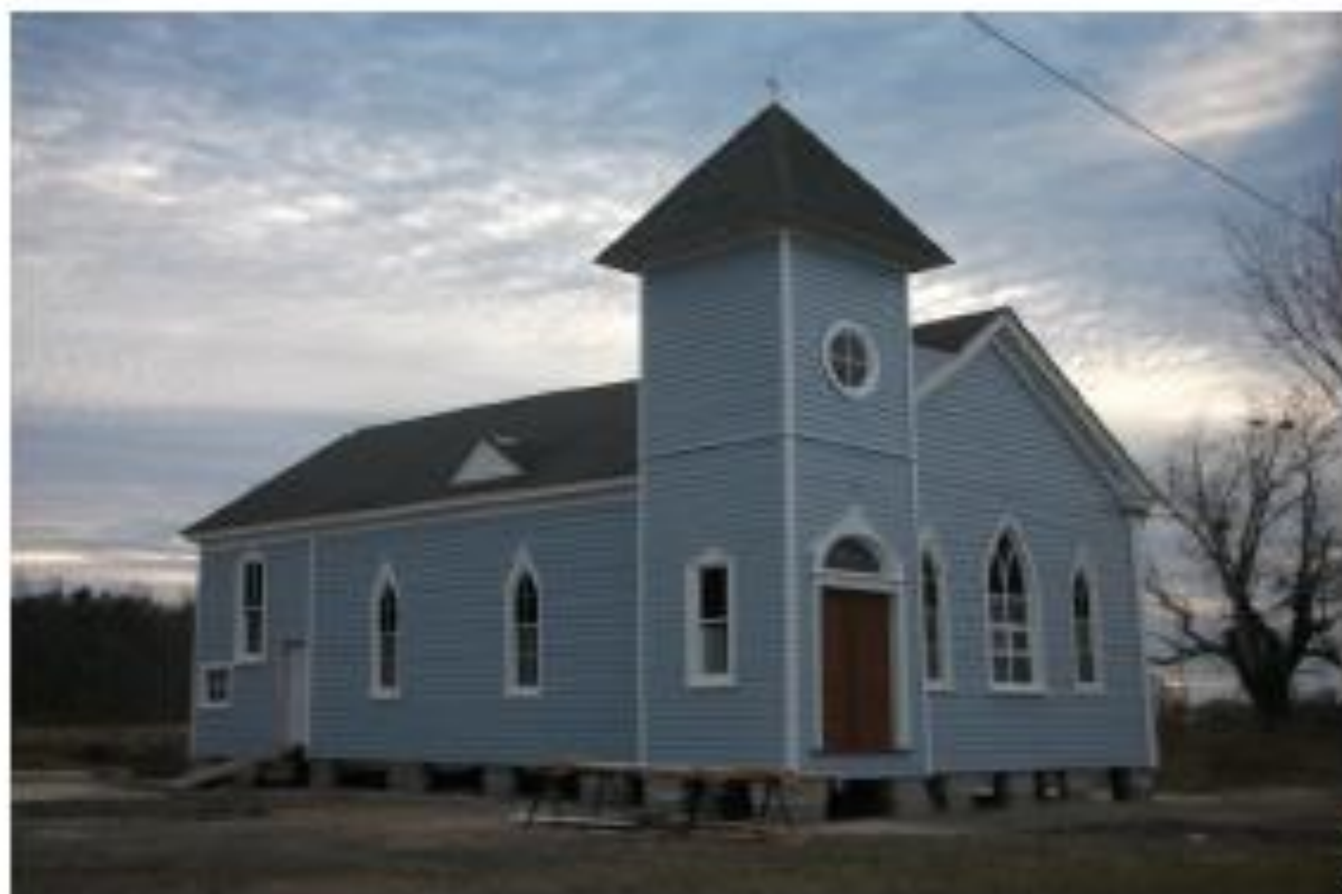
Left: Christ Rock Church after restoration of doors, windows, and siding.
