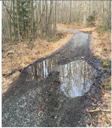
Example drainage remediation site
