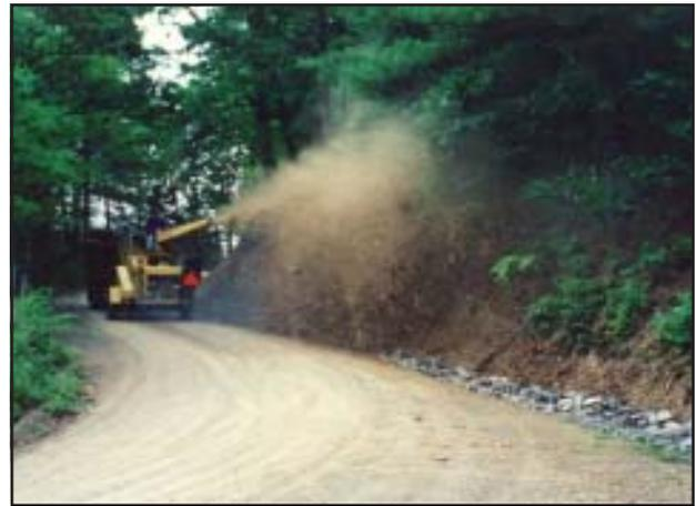
Establishing proper drainage and stabilizing road banks with seed.
