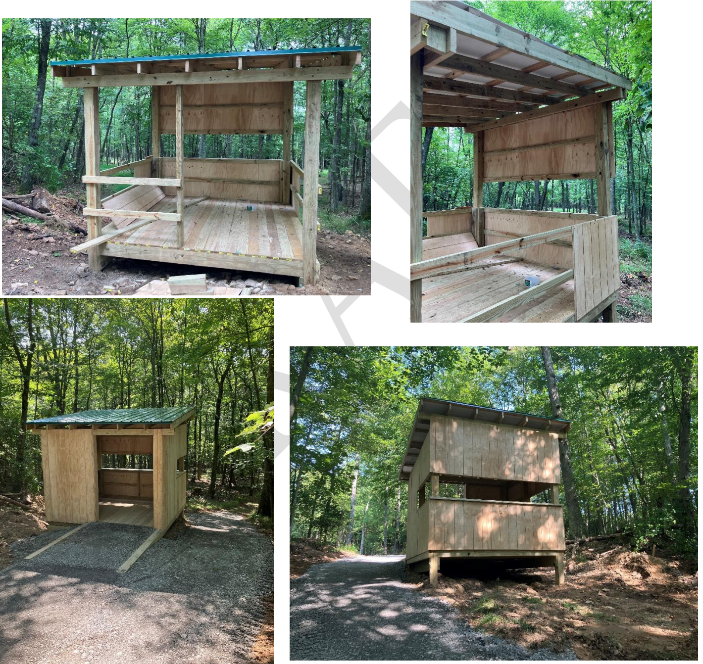
Figure 7. Maple Glade Road Disabled Hunter Enhanced Hunting Opportunity Project construction sequence.
