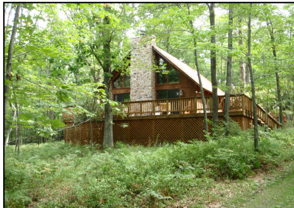
A Wildland-Urban Interface home, with poor defensible space
