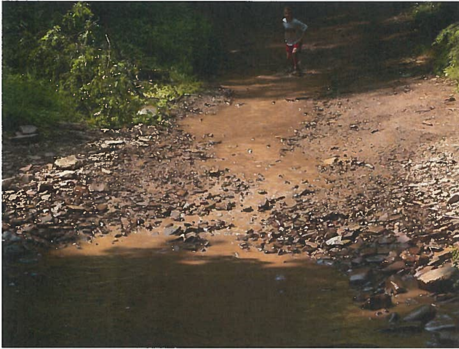
1) Turbid water from an ORV passage running down the road and into the stream.
