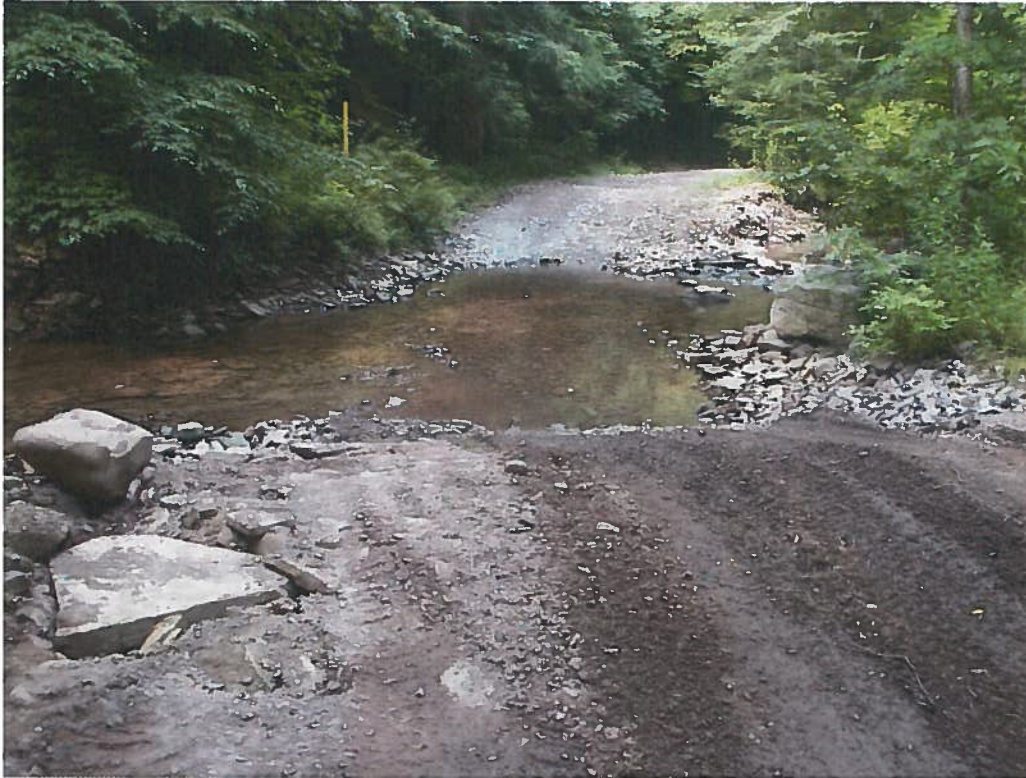
9) Stream channel widening, canopy opening, bank erosion, bare earth runoff.
