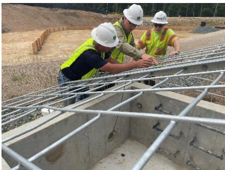
Installing temperature loggers
