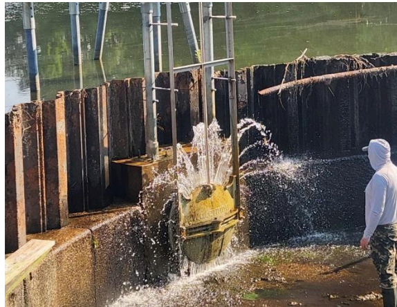
Valve repair at Smithville Lake.
