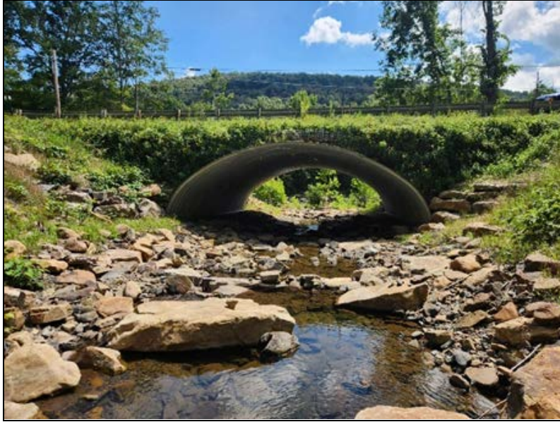
Fish passage friendly bridge constructed over Wolfden Run in 2024.
