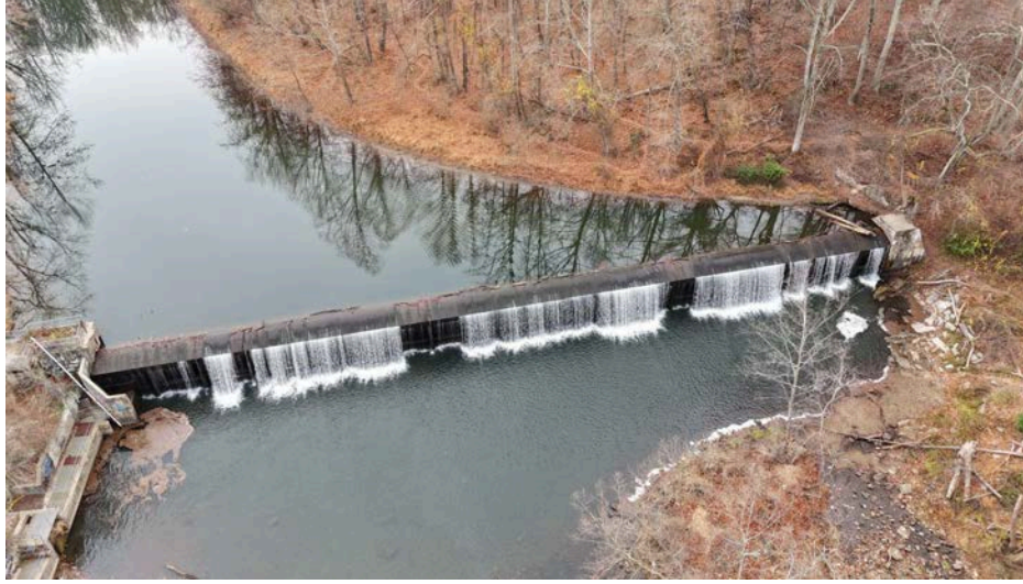
Aerial view of Cypress Branch Dam
