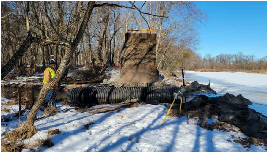
Access road being constructed for the Cypress Branch Dam Removal.
