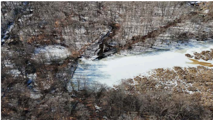
Aerial view of Cypress Branch Dam, impoundment, and access road.
