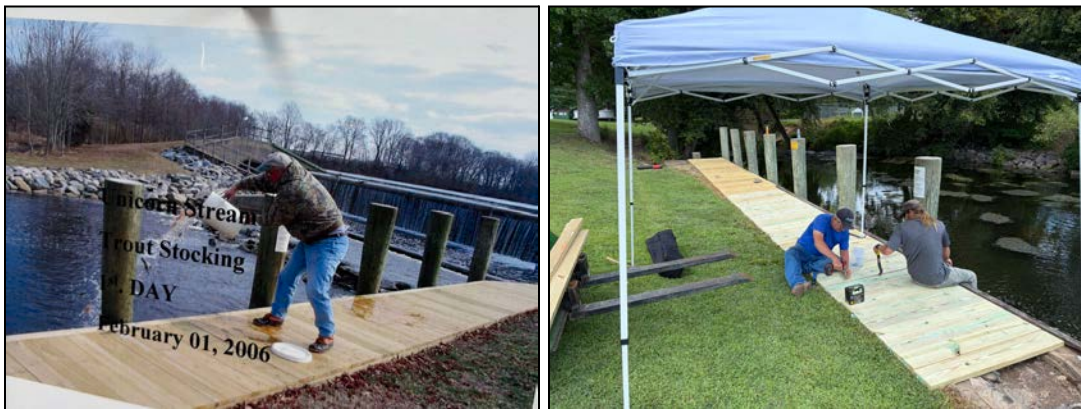
Eastern Regional staff replacing the 20 year-old decking of the bulkheaded section of stream below Unicorn Lake.
