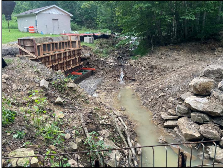
Partial completion of the Winebrenner Run fish passage project. The culverts have been removed and bridge construction has started.
