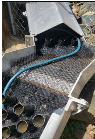
Fish and eel ladder work at Eden Mill Dam
