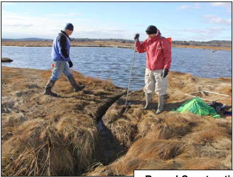
Runnel Construction at Parker River NWR
