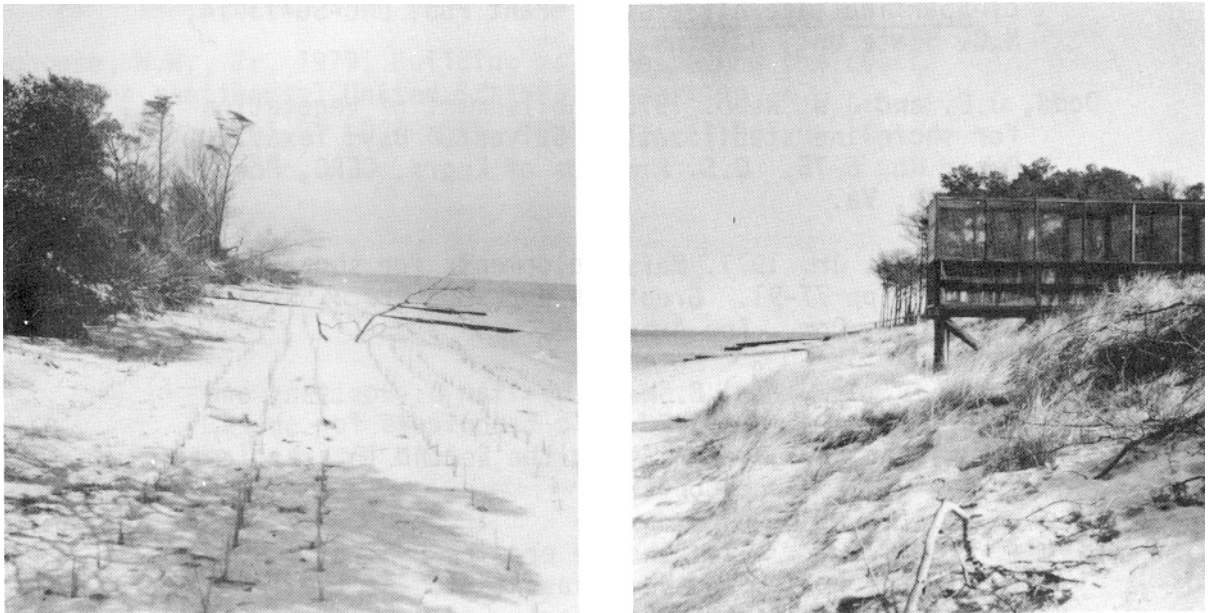
Figure 14 - On the left are groins filled with sand that have been recently planted to American beachgrass. On the right are groins and American beachgrass combined to accumulate sand and tie it into the bank. Note the tips of the jetties sticking out of the water.
