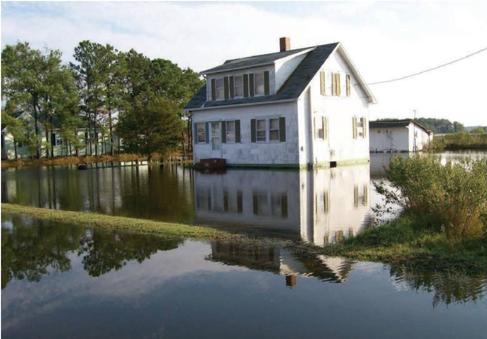
New freeboard standards in Dorchester County, Maryland, can help limit damage to structures when heavy rains and unusually high tides overwhelm existing defenses and cause local flooding as illustrated here. Credit: Wanda Cole
