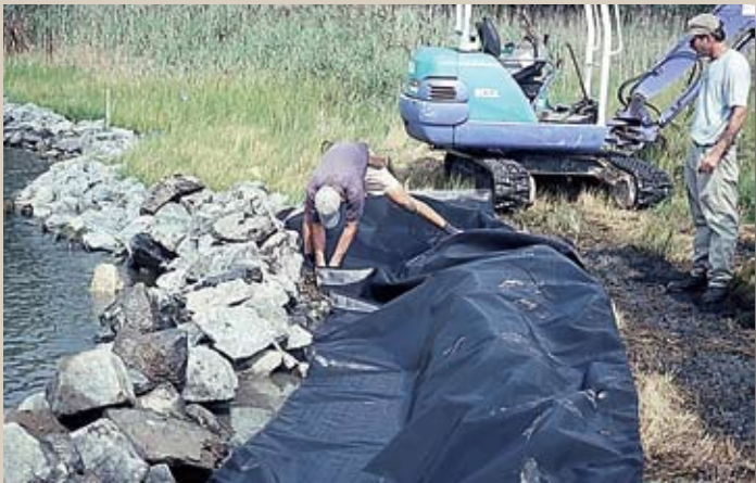
Placement of filter cloth under the stone is essential to ensure project success.
