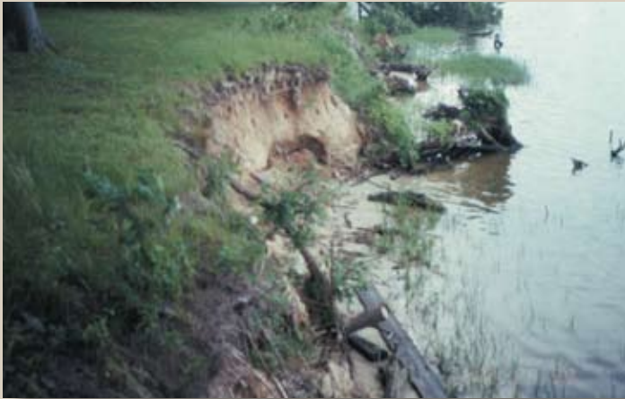
Severe erosion on an 8 foot high unvegetated bank.
