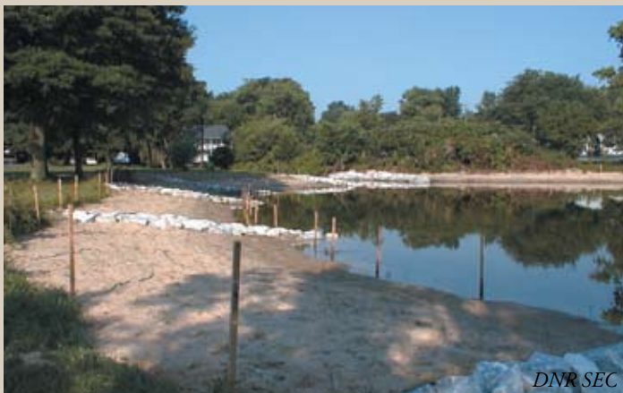
AFTER: Stone groins and marsh fringe constructed to address the erosion problem.
