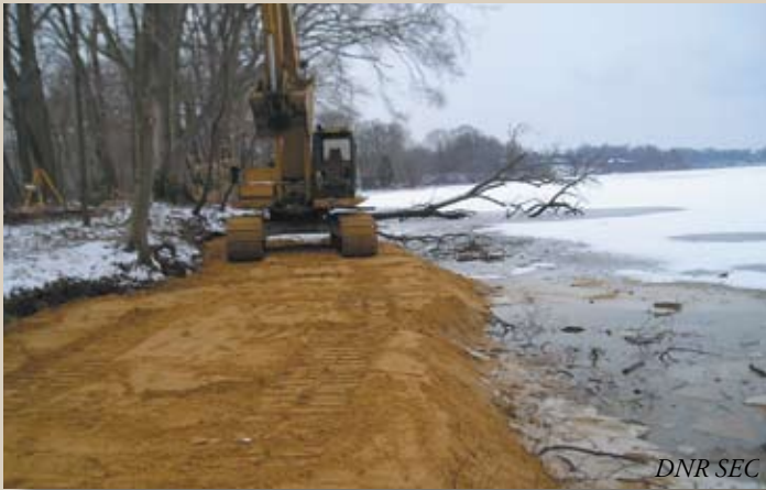
Sand fill is placed and graded to the water's edge.
