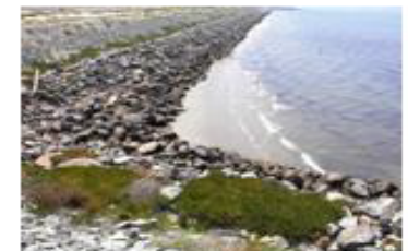
Structural erosion control practice
