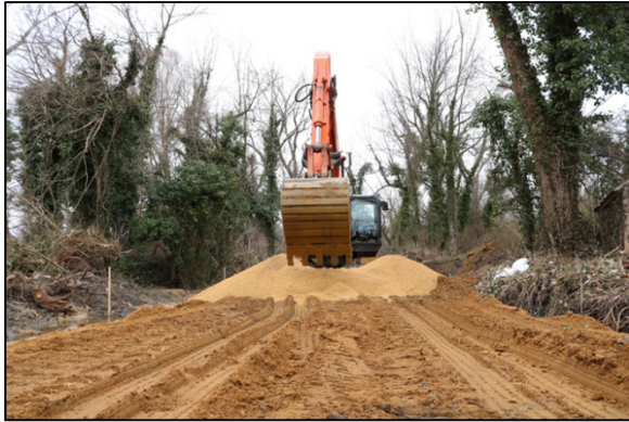
Figure 17. Construction of in stream haul road with sand and woodchip. Contractor backs trucks to the edge, as evidenced by tire tracks, and dumps material in place.
