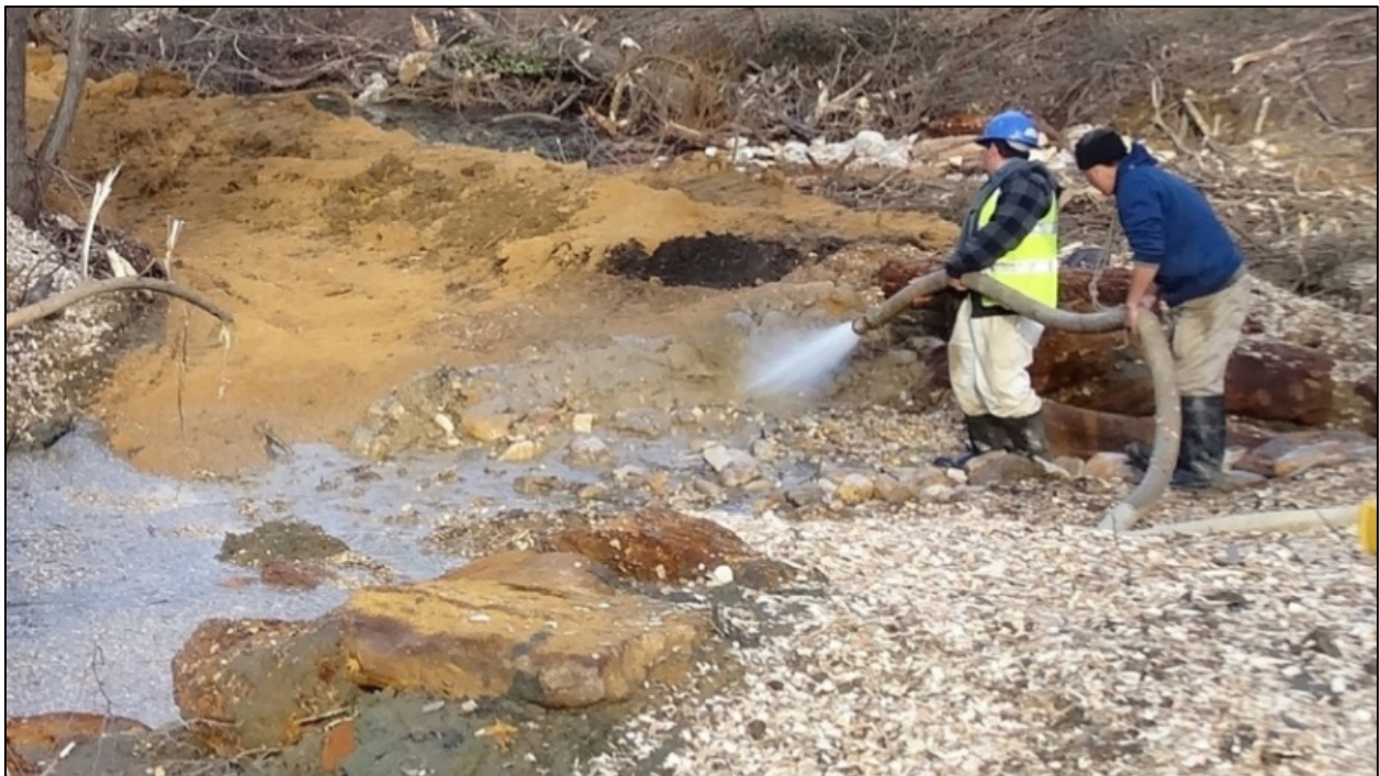
Figure 41. Wash in structures with sand and gravel to fill voids. This should be repeated to sufficiently fill voids, observe flow paths and adjust, if necessary, with more gravel and cobble.
