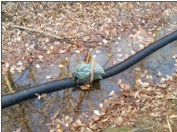
Figure 23. Slotted pipes must be secured with sand bags and stakes to prevent buckling during pea gravel seam installation.
