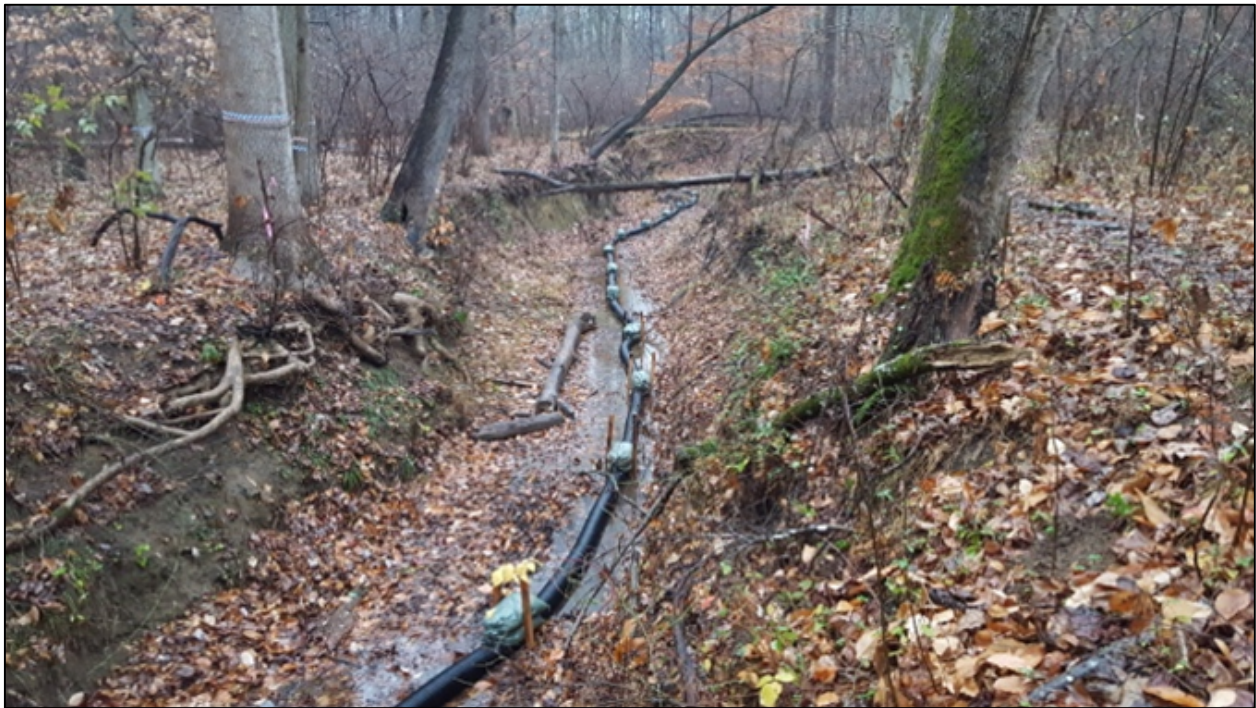
Figure 20. Slotted underdrain system functions as a french drain to help keep haul road dry and convey baseflow during construction. Sections of pipe must be removed during sequential construction of pools to restore surface flow.
