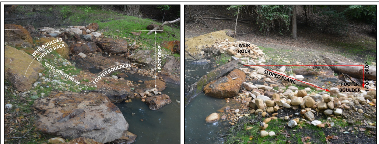
Figure 35. Riffle-weirs constructed with one-foot difference in elevation between the top and bottom edges to avoid sheer drops and safely convey large storm flows. Photo on left is an example of a riffle-weir constructed with weir boulders. Photo on right is an example of a “cobble weir” constructed with footer boulders and river rock (cobble). In both cases, boulders are tilted downstream to convey flow to pool without increased force on stream bed (sheer stress) and a gentle curve is formed to broaden flow.
