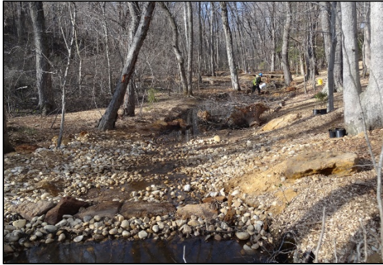
Figure 39. Riffle with scattered erratics extending upstream from weir boulders. Apron of river rock extends downstream from weir boulders and into the pool.
