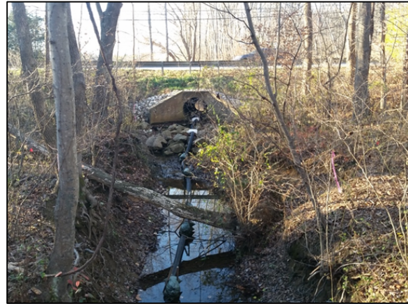
Figure 22. Slotted pipe is inserted into outfall and capped. For large drainage areas, sandbag dikes should be installed sufficiently downstream to create pooling area, as seen in the photo, for clean water diversion.
