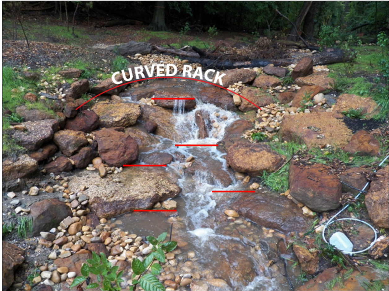
Figure 53. Gentle curved rack spreads flow across the cascade. Flat and alternating placement of boulders breaks flow. Tie in boulders extend into the berm or existing ground with many buried.
