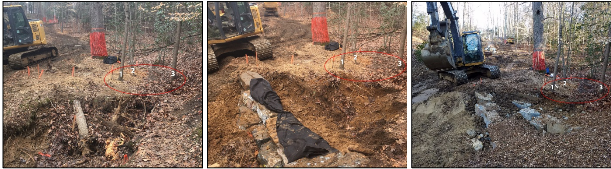
Figure 36. Large trees voluntarily marked with orange construction fencing to avoid removal before haul road construction. Smaller trees saved by the contractor until weir construction before determining need for removal. The contractor successfully constructed the weir per plans without removing the trees (red circles show same trees pre, during and post construction).
