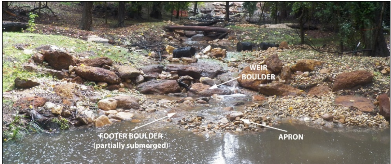
Figure 34. Upstream view of riffle-weir with submerged footer border, apron and weir boulders.
