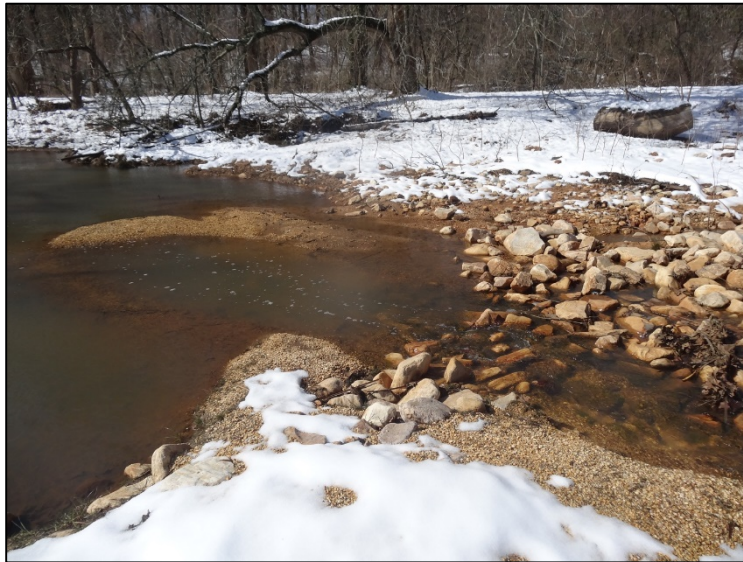
Figure 32. “Cobble weir” with footer boulders submerged and river rocks (cobble) used to hold the grade. It was constructed with sufficient gravel in pools, riffle-weir and along edges to enable formation of diverse flow characteristics, stream bed and habitat.
