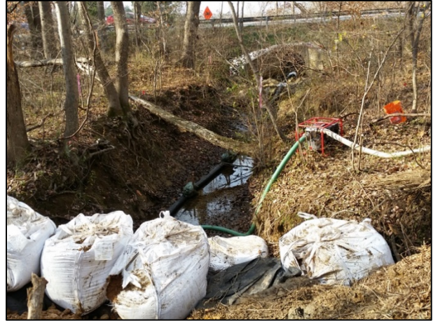
Figure 25. Slotted pipe underdrain must be used in conjunction with a pump around practice that is sized to handle the volumes of the drainage area.
