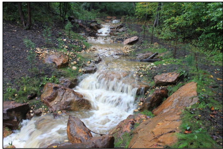
Figure 6. Example of deeply incised outfalls (streams at end of stormwater pipe) that were restored with sand and woodchip filter bed, riffle-weirs, pools and cascades. These are fill projects that raise the stream bed to reconnect with the floodplain.
