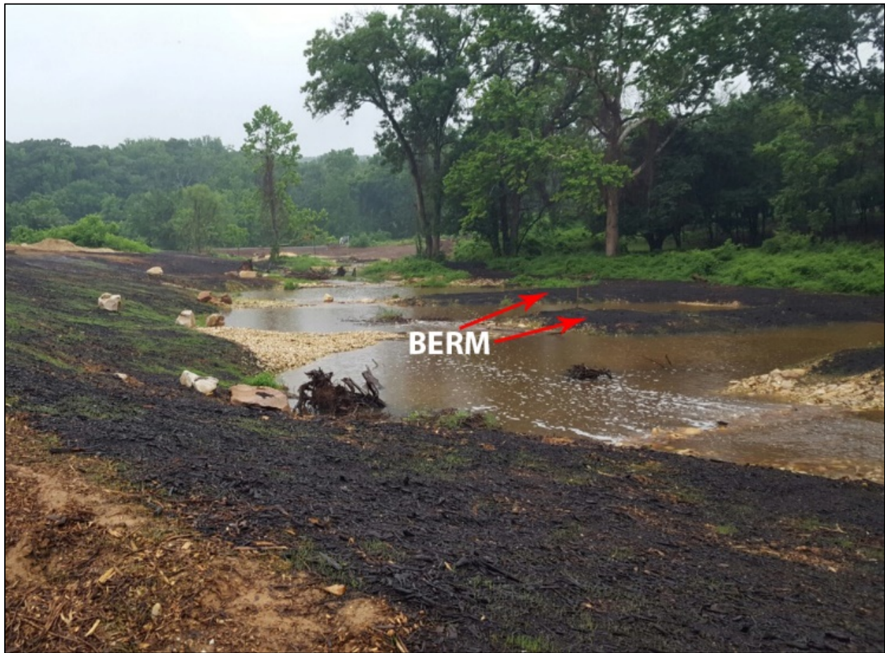
Figure 45. Berms holding water to keep flow from cutting around the weir, spreading water out, increasing exchanges of surface and groundwater and filtering water through their medium.
