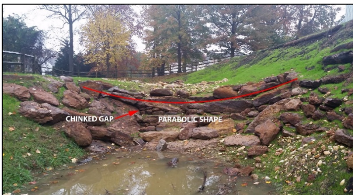
Figure 51. Subgrade is excavated to support a parabolic shape necessary to keep flow in the center and shoulders. Boulders are placed flat to create falls from top boulder to next rather than continuous surface in a chute. Gaps between boulders have been filled by hand-placing smaller boulders and rock (chinking) in a manner that maintains the general line of the boulders. Range of gravel and cobble sizes have been randomly cast throughout the cascade to allow self-organization throughout time. Spaces between boulders are planted and seed is cast over entire structure to stabilize and naturalize over time.
