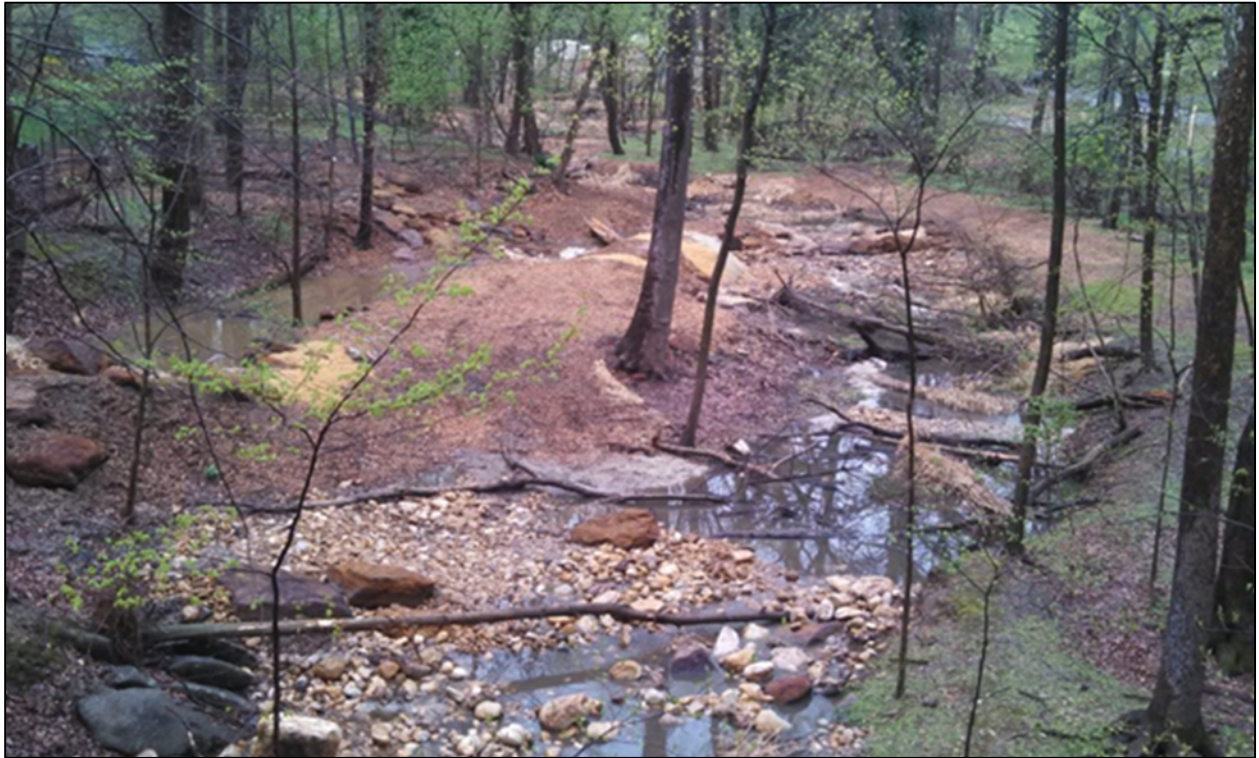
Figure 15. Both larger and smaller trees are left in place during the construction of the haul road and iteratively removed or incorporated into the project during weir and pool construction. Trees removed during construction are used as coarse woody debris in addition to imported stumps, logs and branches.
