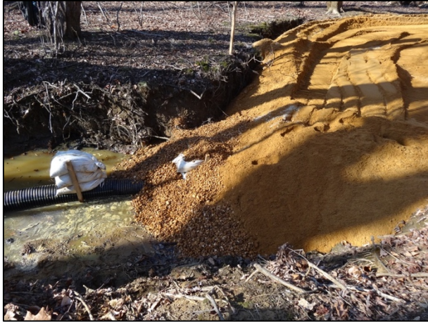
Figure 24. Placement of pea gravel seam over secured slotted pipe and construction of sand and woodchip haul road over the underdrain.
