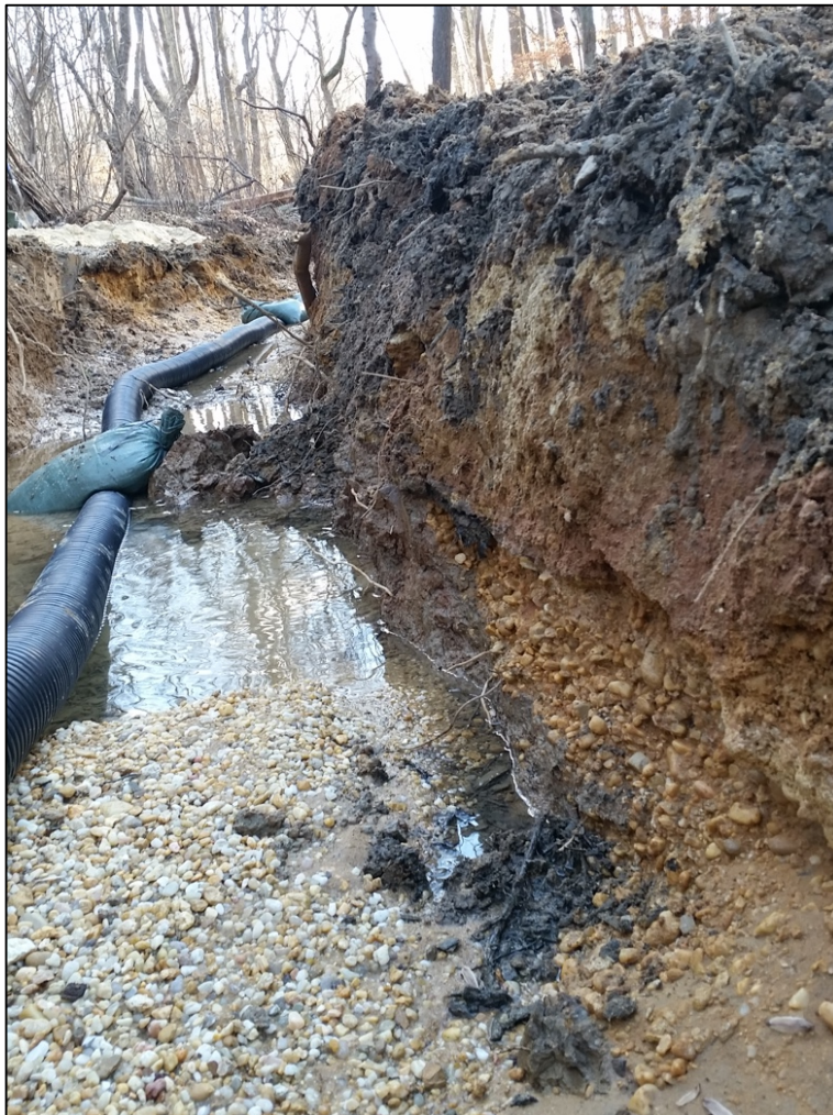
Figure 29. Installation of pea gravel under-drain and seam starting to connect to the native gravel seam (darker gravel on the right side of photo beneath the layer of soil) that has been broken and exposed by bank erosion.
