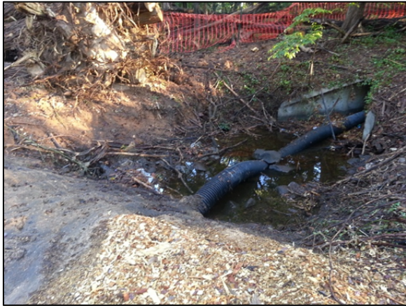
Figure 21. Slotted pipe is inserted into pipe and capped. For smaller drainage areas, haul road can begin immediately downstream as seen in the bottom left of photo. Small pumps can be used to dewater if necessary.
