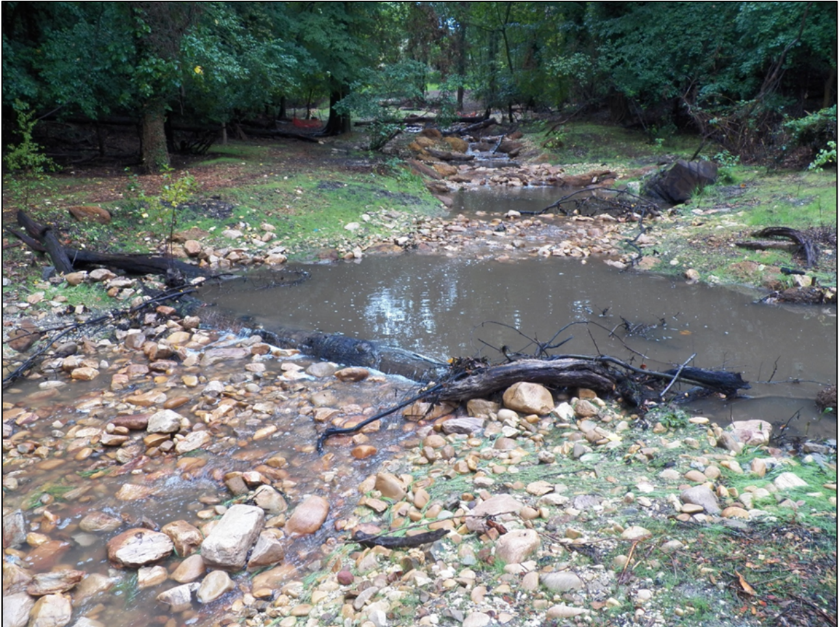
Figure 54. A pool that was widened to further dissipate energy. Edges supplemented with gravel and river rock to create roughness, support diverse geomorphology and provide habitat.
