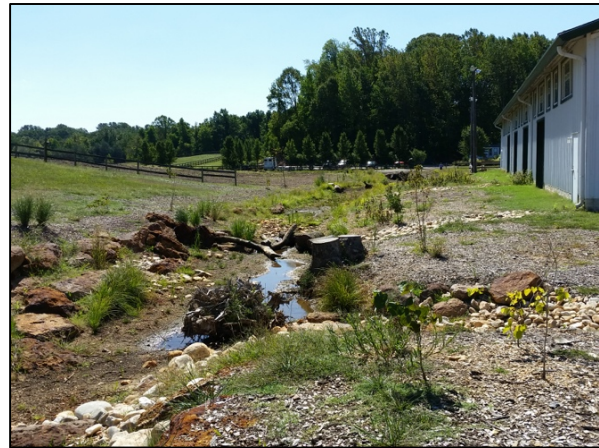
Figure 4. Example of a step pool stormwater conveyance capturing water from rooftop and surrounding fields with compacted soils to filter through sand and woodchip chamber before stormwater drains into a fragile freshwater bog. This was an excavation project.
