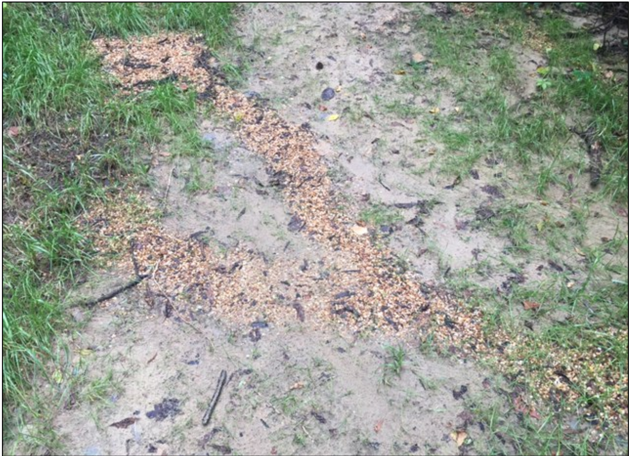
Figure 57. Rills filled to grade with pea gravel to allow water flow to continue in the path it has carved into the newly constructed landscape.
