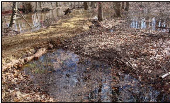
Figure 13. During haul road construction along the edge of the stream, this contractor minimized the width, avoided tree removal and preserved the existing depression on the floodplain (wet areas at the bottom and right side of the photo). Clean sand was used to bridge the haul road across the depression to allow drainage and the depression was not filled or levelled to preserve a diverse topography. Logs were used to keep sand from spilling into the depression, which was kept intact throughout and post construction as seen in the next figure.
