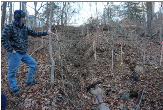
Figure 7. Example of a steep gully and exposed utilities restored with a step pool stormwater conveyance to capture stormwater (flowing down boulder) at the end of a dead end street and non-erosively convey and improve water quality before it enters a stream.
