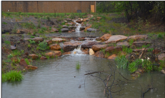
Figure 5. Example of a dry pond retrofit that created sand and woodchip berms and filter beds to increase time of stormwater detention and decrease volume and velocity entering the stream immediately below. This was a fill project.
