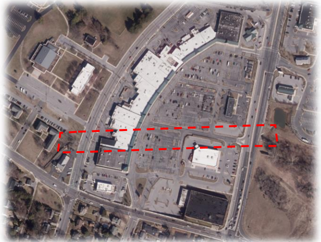
Figure 9: Approximate Location Longmeadow Culvert
