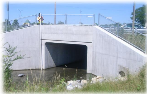
Figure 10: Existing Longmeadow Box Culvert
