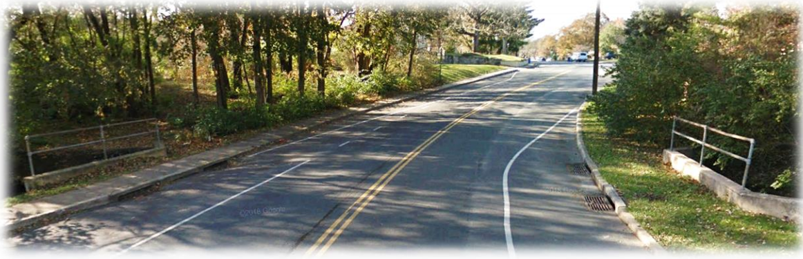
Figure 17: Street View of Magnolia Culvert
