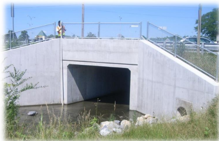
Figure 6: Longmeadow Shopping Center Culvert
