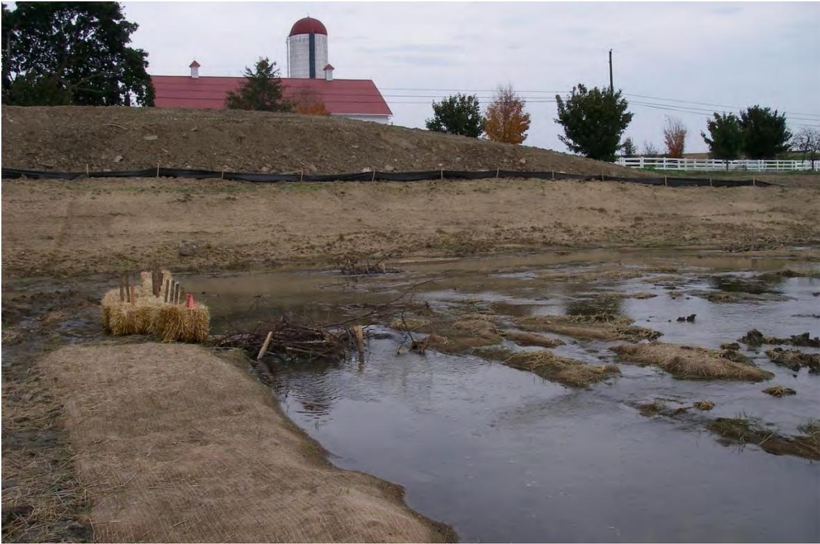
Straw bales to create backwater and increase deposition and reduce further erosion
