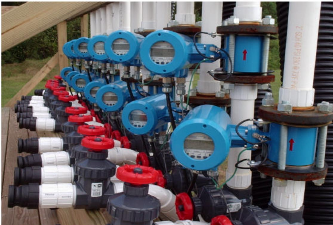
The flowmeters selected for use in the study were the Kronhe Model IFS 1000 Wafer Style Flowmeter with the Model IFC 090 Converter. This type of flowmeter was selected for the following reasons:
