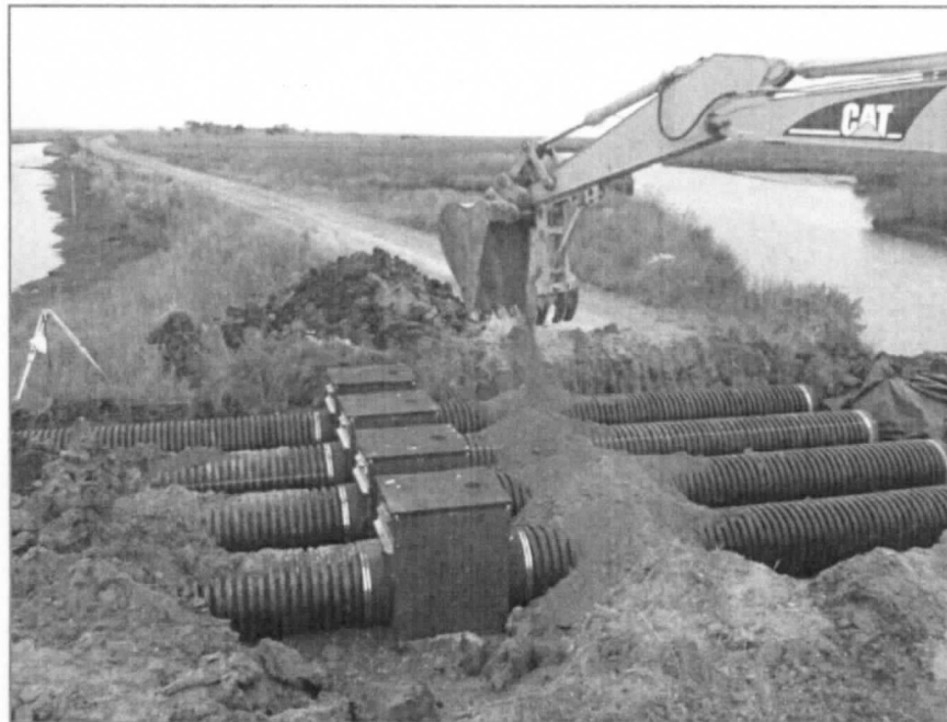
Above: One of two large piling and plank water control structures at Deal Island impoundment. Below: Four in-line water control structures being installed.
