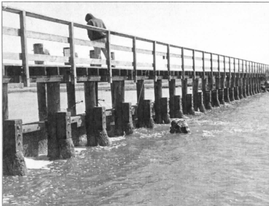
Above: One of two large piling and plank water control structures at Deal Island impoundment. Below: Four in-line water control structures being installed.
