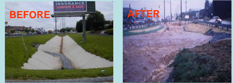
Longwell Branch, in Carroll County before and after a rain storm.
