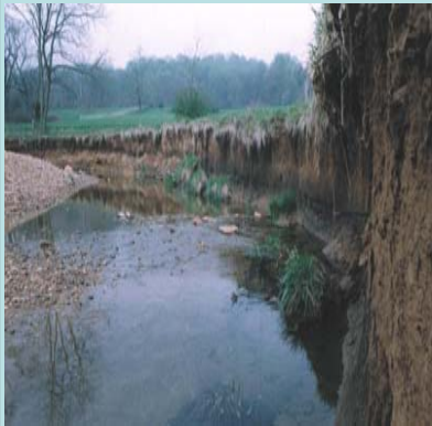
Severe stream bank erosion in Minebank Run, Baltimore County .
