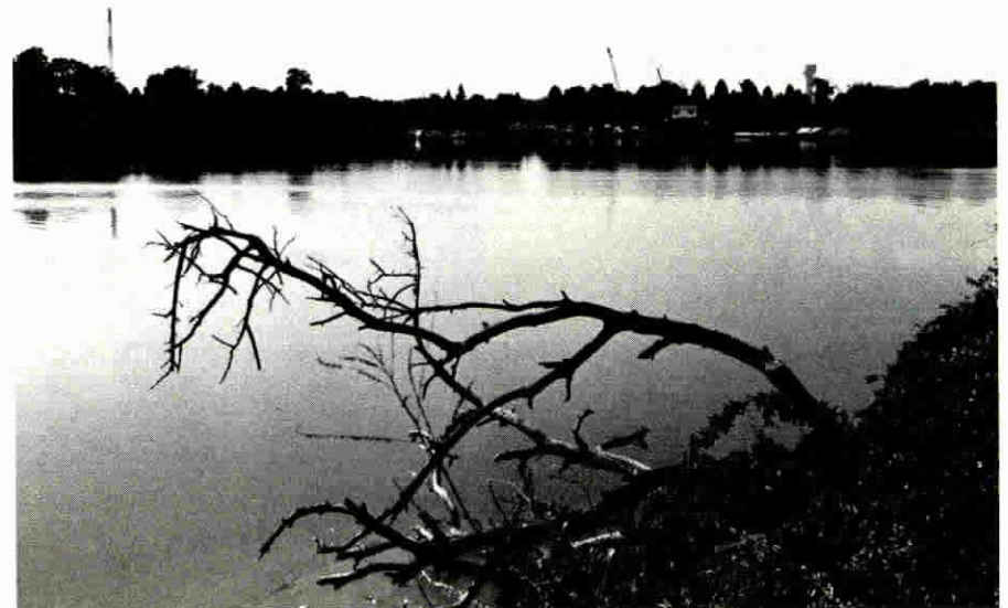
Looking across the Back River at the Baltimore Sewage Treatment Works
