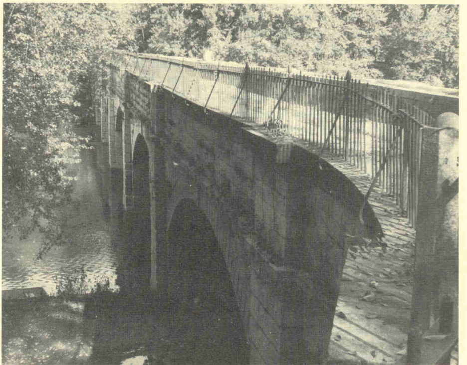
Monocacy Aqueduct - Courtesy of C&O Canal National Historical Park
