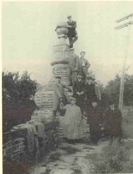
Frederick County - Old Jug Bridge
