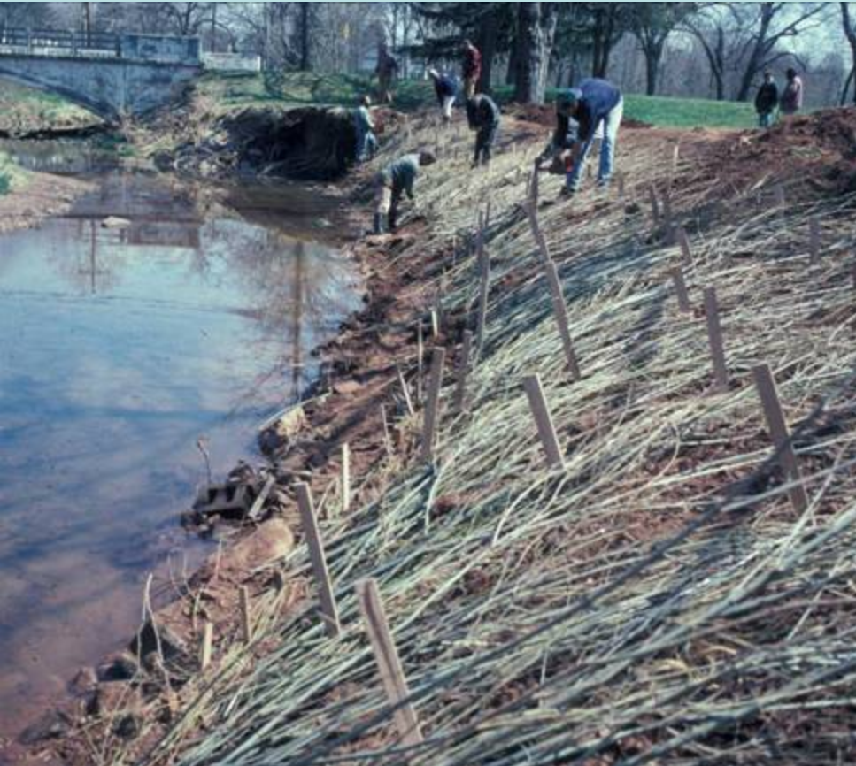
Installation of brushmattress
