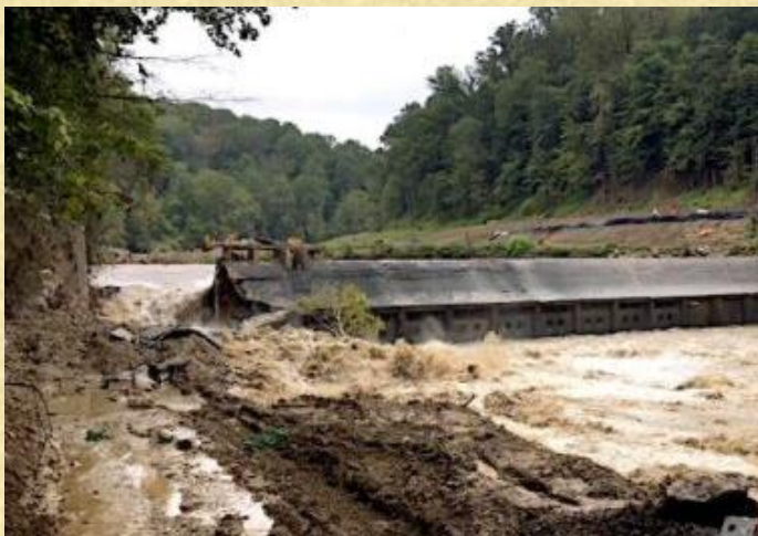
Bloede Dam at Patapsco Valley State Park
